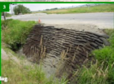
Backfill existing soil into GTX Bag & laying Standard Units between GTX Bag
