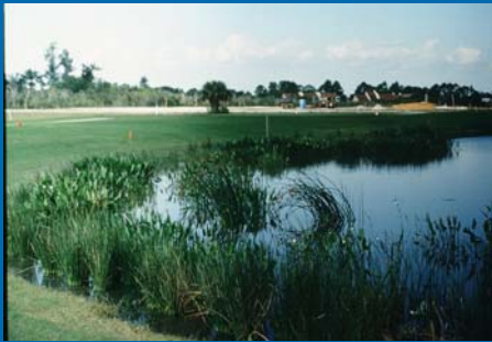
Created Wetlands (Littoral Zone) in Surface Water Management System
