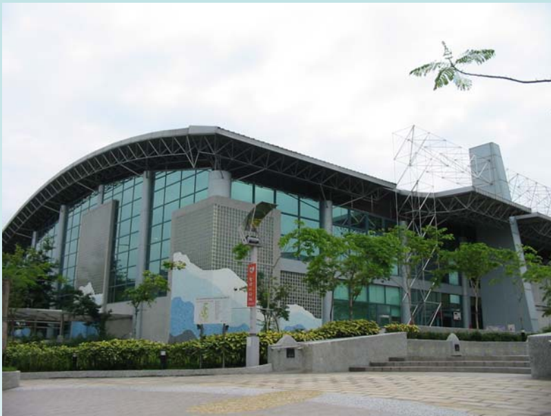
Warm Water Swimming Pool
