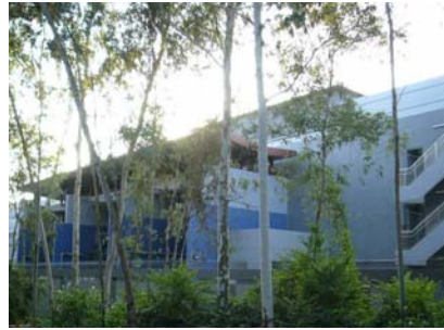
Figure 6. Maintain Trees Around Substation Building
