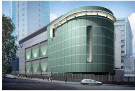
Figure 5. 'Blend-in with Environment' of a 132 kV Substation in Urban Area
