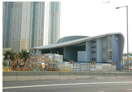
Figure 3. 132 kV Substation Building adjacent to LPG Filling Station
