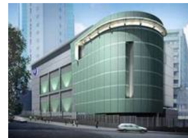
Yiu Wing Street Substation
