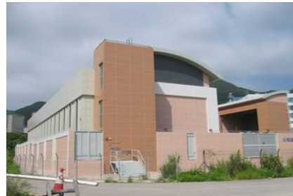
Wan Po Road Substation
