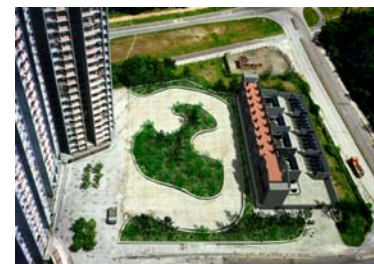
Visual impact - from roof of adjacent estate building
