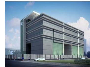
Lai Cheung Road Substation
