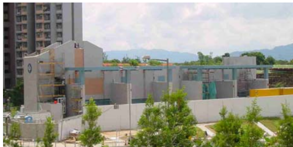
Substation Completed & Commissioned
