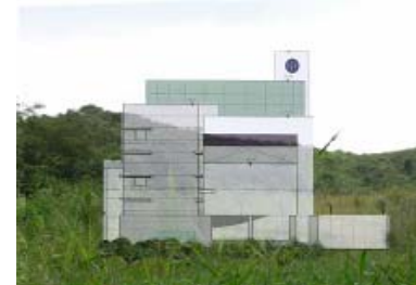
Ma Wan Substation
