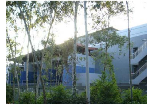
Maintain Trees Around Substation Building
